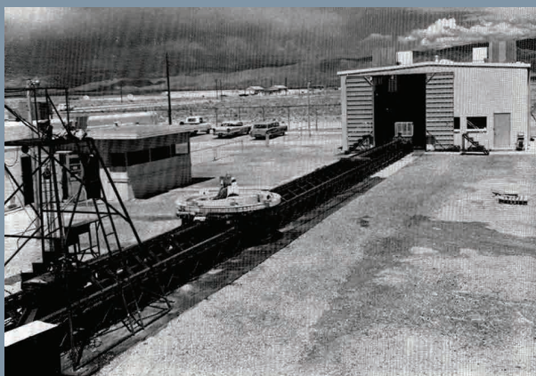
Colonel Stapp's Daisy Decelerator at Holloman Air Force Base. This view captures a human run in an omnidirectional sled. The airgun accelerator mechanism was housed in the building to the right. The tower to the left held high-speed cameras. (U.S. Air Force)
