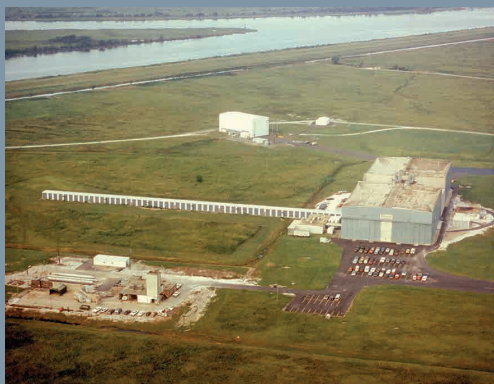
The enclosure for the horizontal impact accelerator's 700-foot-track extends into the marshy area outside building 420 at Michoud. (USAARL)
