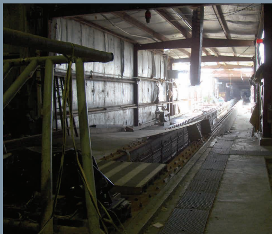
Damage to the horizontal accelerator building enclosure caused by Hurricane Katrina. (USAARL)
