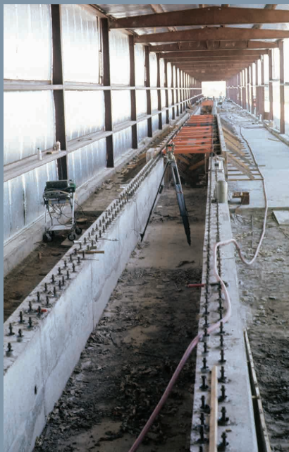
Left: Construction continues on the enclosure and foundation for the long-track horizontal impact accelerator. (USAARL)
